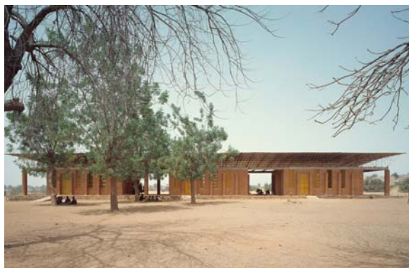
Figure 4: Gando Primary School
