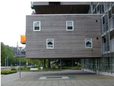
Steel trusses make dramatic cantilevers a possibility in MVRDV's WoZoCo building.
