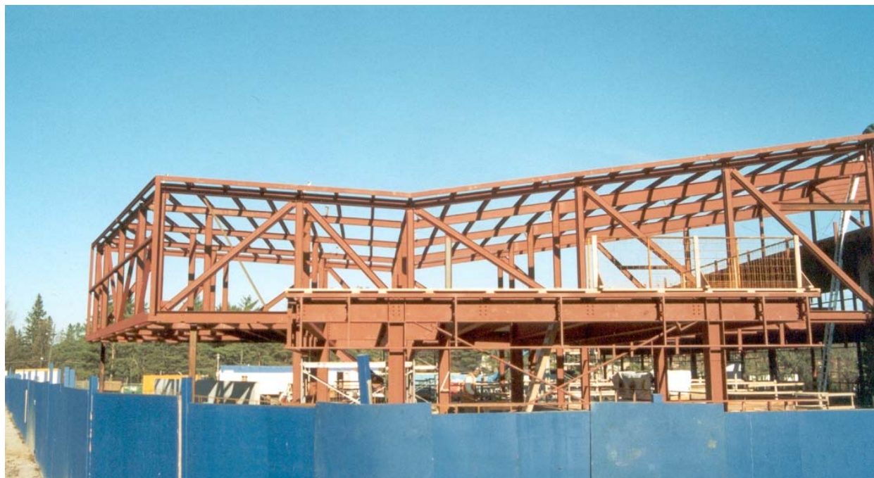
The Royal Ontario Museum - top - is getting stripped of its steel girders so they can be reused at the University of Toronto Scarborough Student Centre - bottom.
