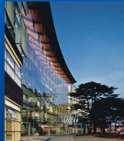
Fingal County Offices Bucholz McEvoy Architects
